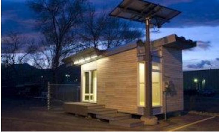
*CU Denver architecture professor Julee Herdt built this structure out of her BioSIP system, super strong boards made of 100 percent recycled material. Credit: University of Colorado Denver*
